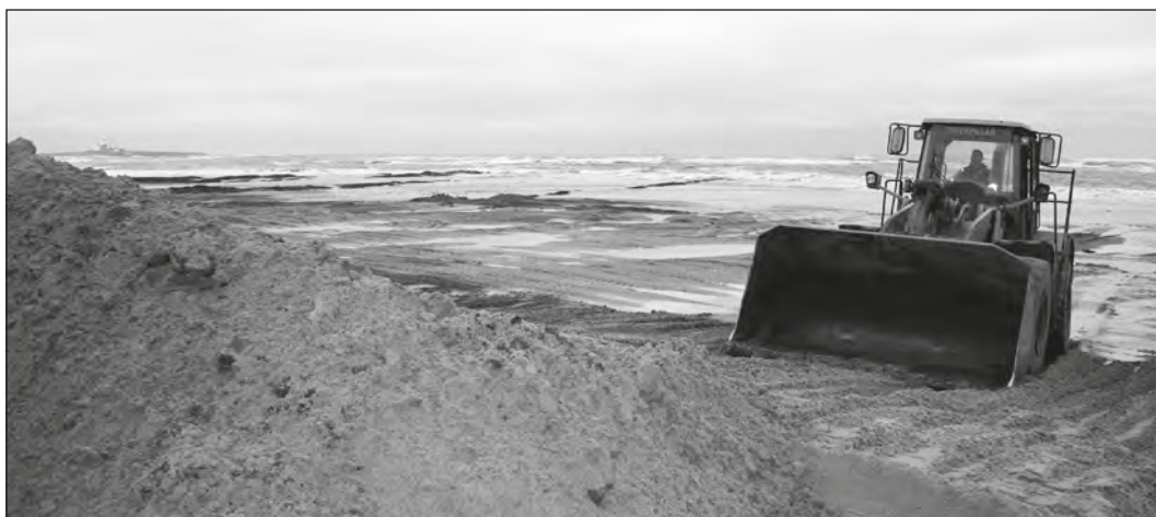
Above: a digger moves sand to the foot of the dunes in emergency repair work at Low Hauxley
