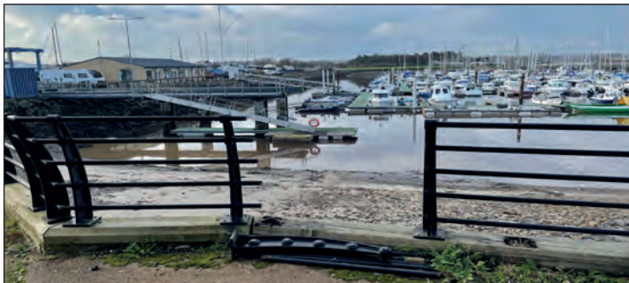
A section of the railings has been removed and some bolts have become loosened along the walkway
