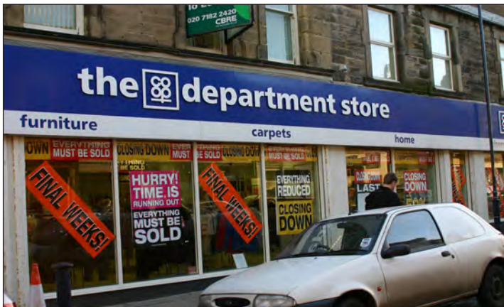
The Co-op department store closed in 2006. The building now houses shops, a restaurant, and flats above.
