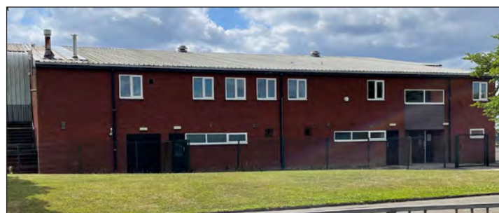
The old sports hall at JCSC is destined to be demolished unless NCC agree to a Community Asset Transfer
