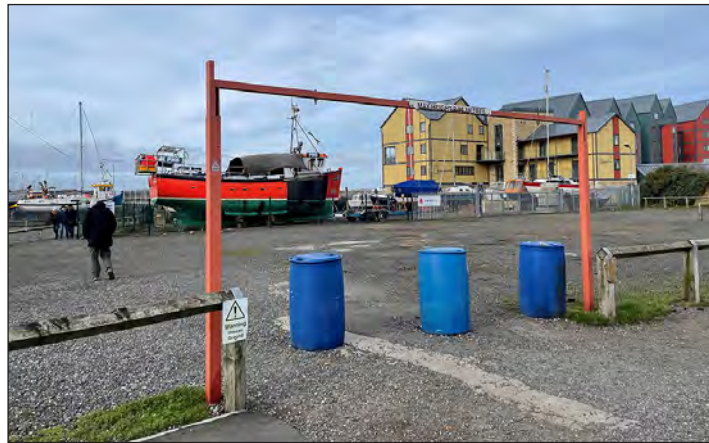
A complex land deal between NCC and Amble Marina needs to be finalised before work on the walkway can commence
